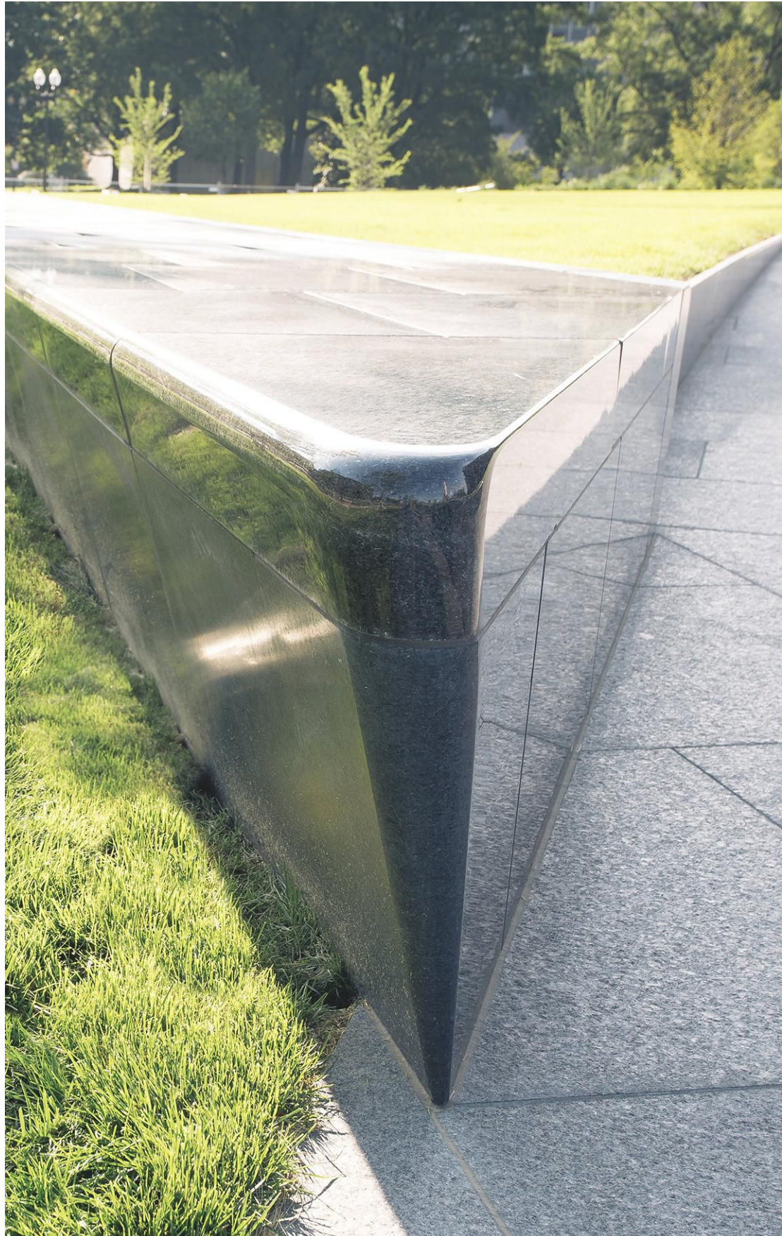
The pathway up on the north side takes you past massive trapezoids of black granite bollards topped with bullnose corners, a design detail that kept the team on its toes. Photo courtesy of DC Real Estate
